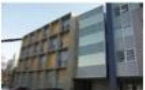
Bench Scale Facility
