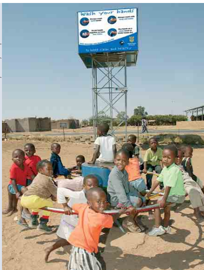
An hour's play produces up to 370 gallons of water. The billboards carry public health messages and generate advertising revenue to fund maintenance.
