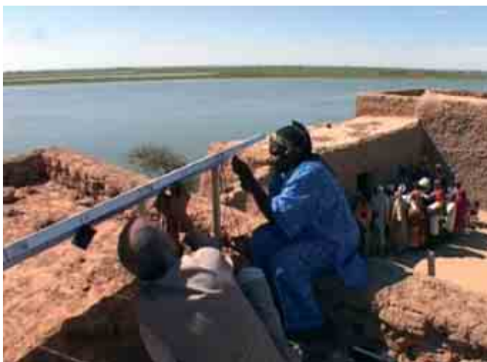
Installation of solar panels in the village of Dejegalia, Timbuktu, Mali
